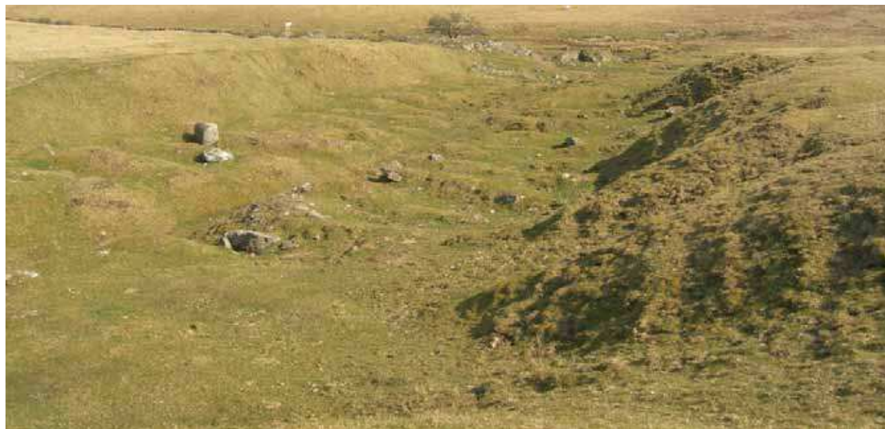
Figure 6 Eluvial streamworks in the dry valley between Leskernick Hill and Bray Down on West Moor, Bodmin Moor. Reservoirs on the far side of the cutting stored water for use in the tyes, on the nearer uphill sides of the parallel dumps that lie each side of the central drain. Leats brought water to the tyes on the nearer side. Three tinner's lodges or shelters survive at the sheltered far end. See Sharpe 2008, fig 32 for a survey and interpretation of this site. Further streamworks can be seen in the distance (top right). (Photo: Peter Herring).
