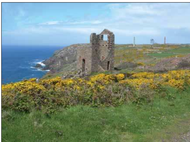
Figure 18 The Wheal Edward stamping engine's house, was part of the Wheal Owles mine in St Just at the time of a terrible disaster in 1893 when 20 men drowned as miners broke through to flooded older workings. (Photo: Peter Herring)
